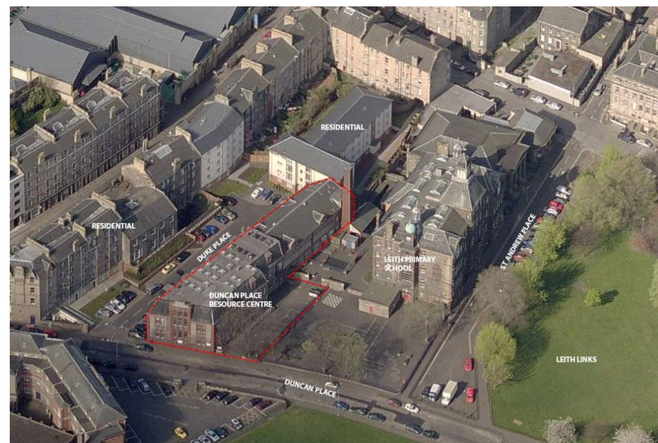
Figure 3 - Aerial view of Duncan Place Resource Centre Facing North.
